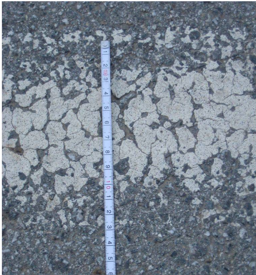
Figure 3: A photograph (26 Mar 2008) showing a measurement of the roadway stripe with a cm scale showing 14 cm width (5.5 inches), taken on the Woodside side of the town line.
